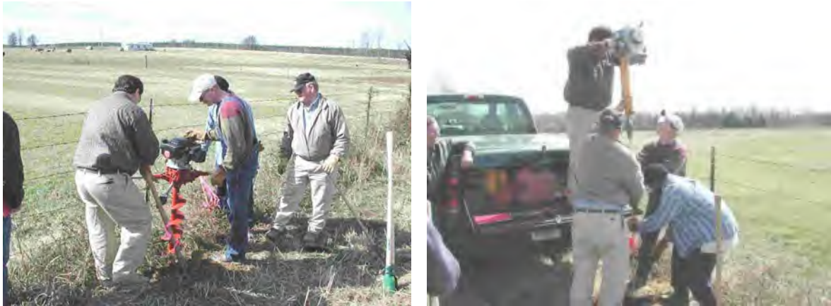
Figure 8-11. Setting deep-driven bench marks (Memphis District & 3001, Inc.)
